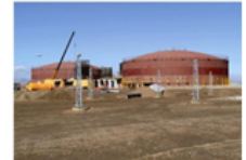
Salt Tanks for Thermal Storage
